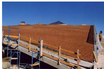
After the substrate layer was applied.
