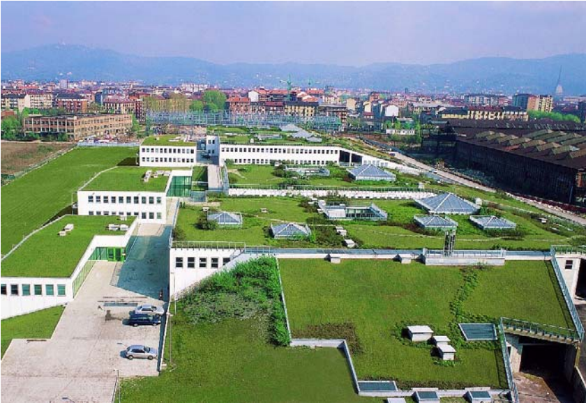
The flat and pitched green roofs of the Environment Park.
